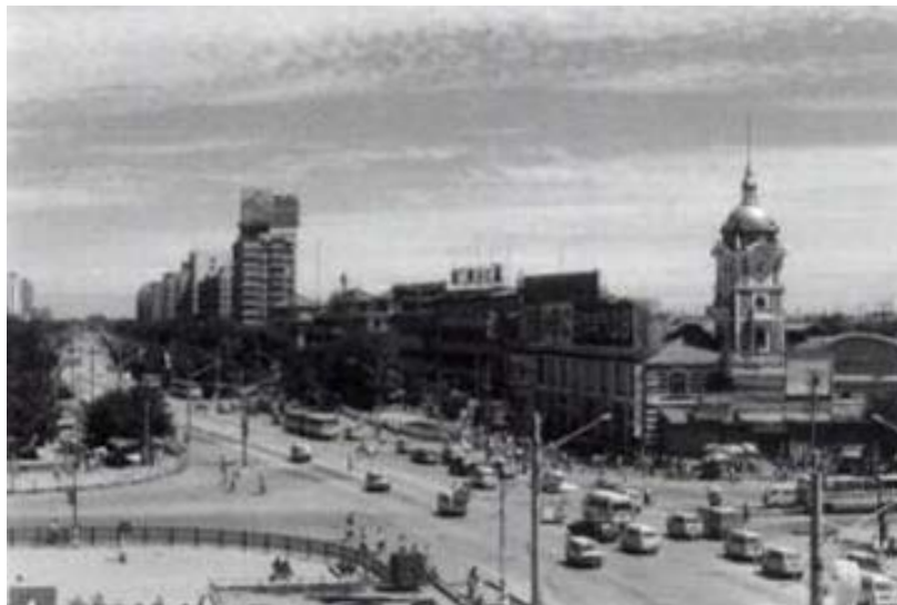
Figure 2 – Clock tower atop the Qian Gate Rail Station 51
